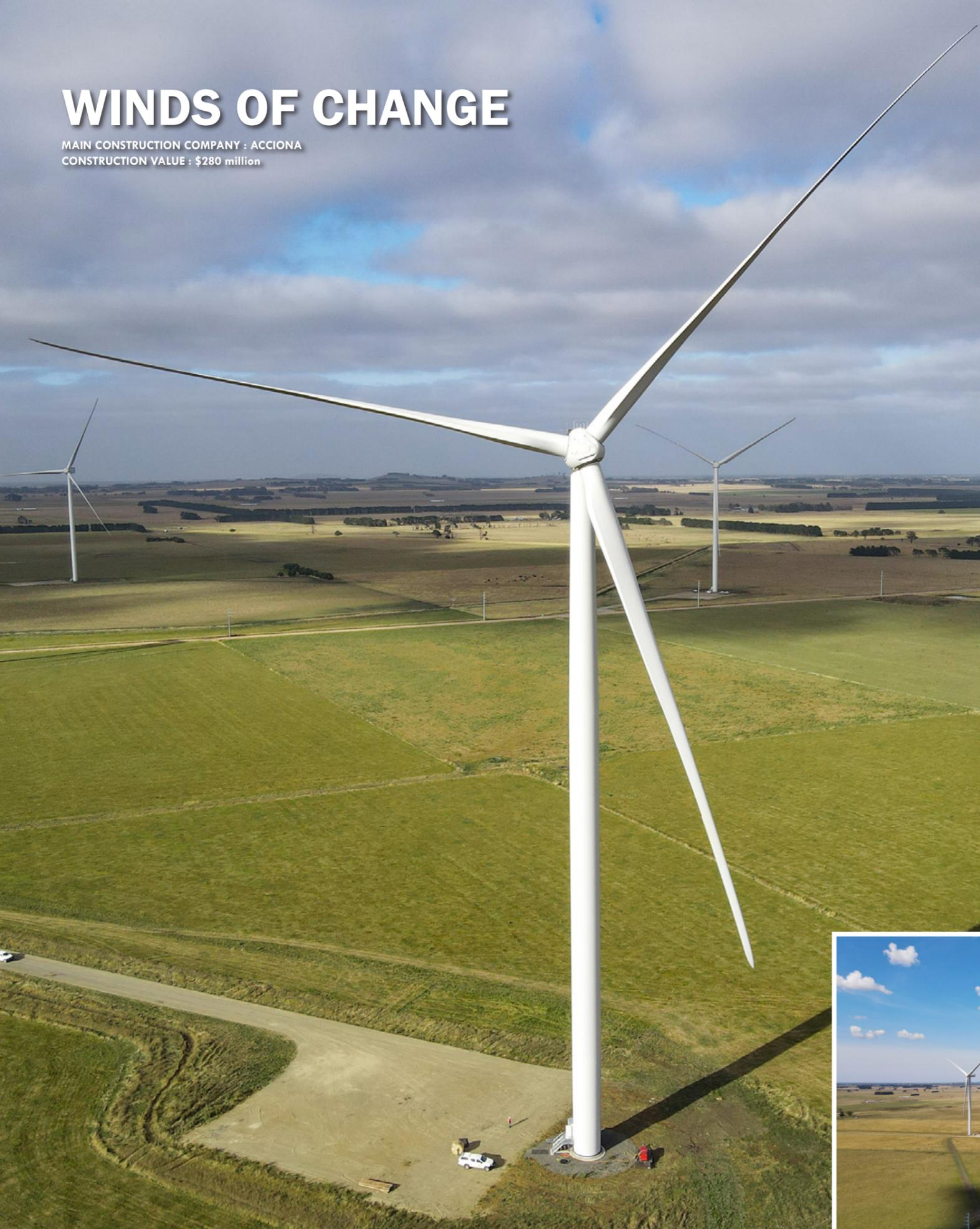
Mortlake South Wind Farm includes 35 Nordex 4.5MW turbines with a capacity up to 157.5 MW, which will generate clean energy for the equivalent of up to 117,000 households and a 15km underground connection line to the 220kV Terang substation. The wind farm will assist the Victorian Government's target of 40% of electricity generation from renewable sources by 2025, while bringing significant economic activity to the region.
