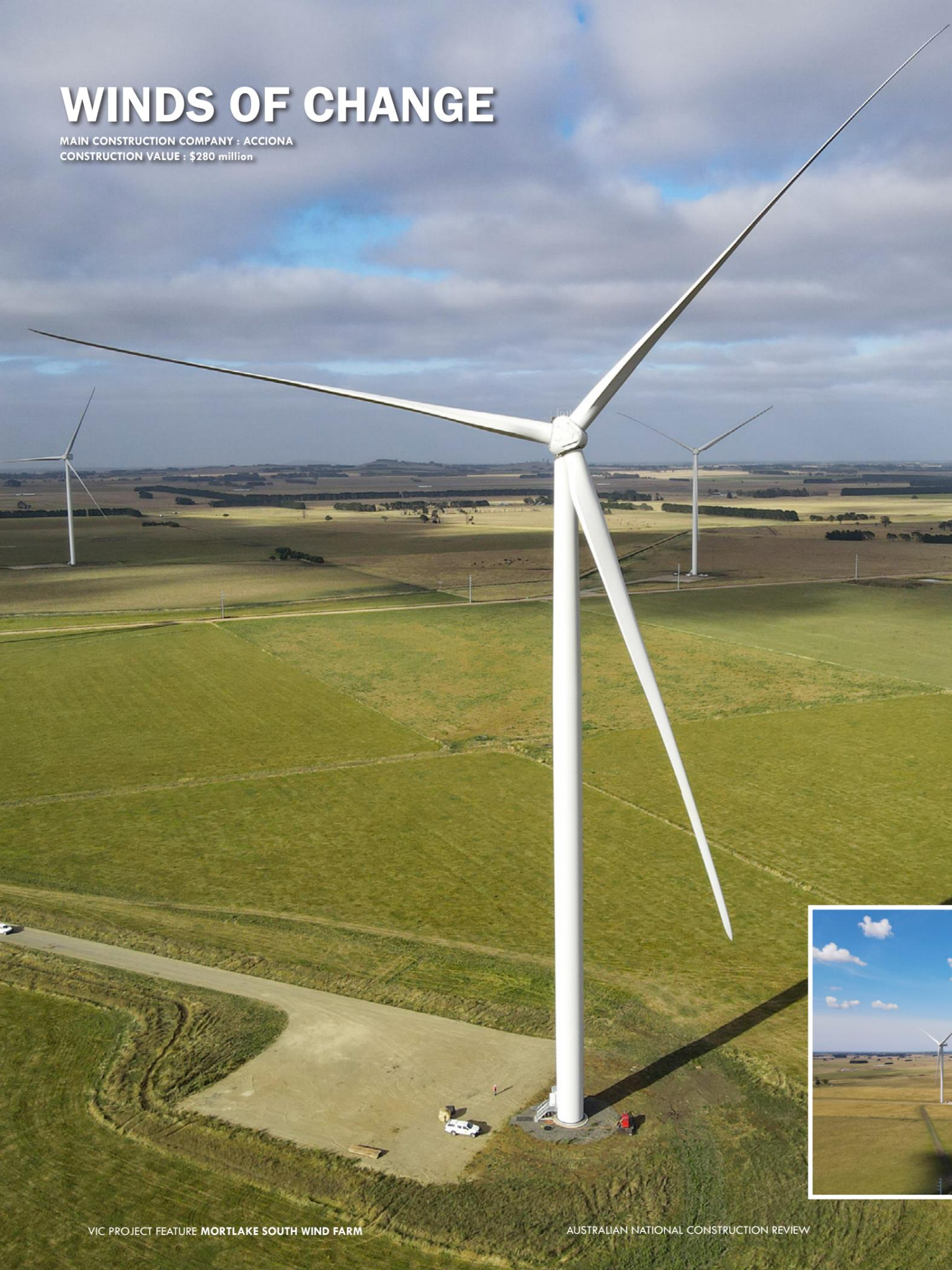
Mortlake South Wind Farm includes 35 Nordex 4.5MW turbines with a capacity up to 157.5 MW, which will generate clean energy for the equivalent of up to 117,000 households and a 15km underground connection line to the 220kV Terang substation. The wind farm will assist the Victorian Government's target of 40% of electricity generation from renewable sources by 2025, while bringing significant economic activity to the region.
