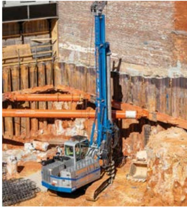
"Drilling in extremely high strength rock is not uncommon for Canberra," said Canberra Drilling Rigs', Dale Gaffey. "We beat this by using great tooling to cut through the rock, in particular, using the correct drill bits got us through."
