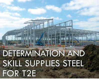
ith 2,300 tonnes of structural steel to supply, fabricate and install for the T2E project, Aus Iron Industries expanded their own capabilities, implementing new micro-management processes and investing in new capital technology. Aus Iron provided both the structural steel for the two new gates at Melbourne Airport, and for the new baggage handling facility.
