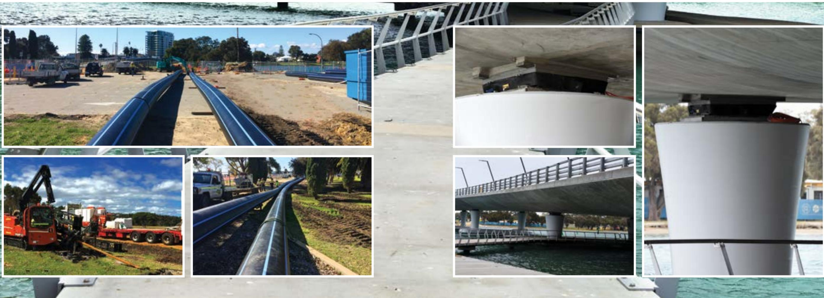
Specialists in directional and vertical drilling, Power On Cabling were chosen to lay the gas and water pipes for the Mandurah Traffic Bridge Replacement project. Unlike the old bridge, the utility pipes do not run alongside the structure, instead they sit deep within the river bed. Power On Cabling were the only company in the state with the right expertise and equipment to drill under the estuary.
