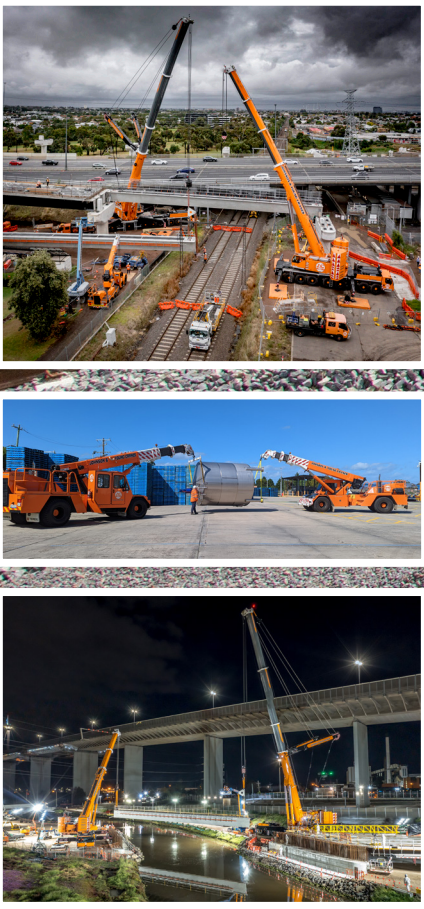
A Pedestrian Bridge being lifted into place at the Frankston line.
