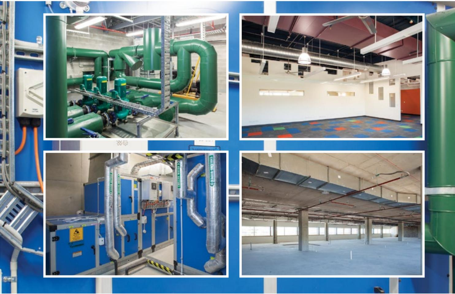
For a university located in the tropical environment of Townsville, keeping both indoor temperatures and also energy consumption down is vital, which is why RST Air Conditioning delivered a unique design for the JCU Clinical Practice Building, which uses the university's existing chilled water ring main to cool the air.
