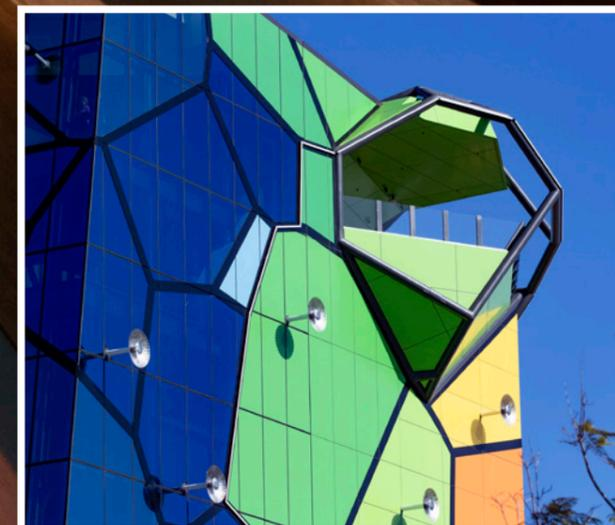
The stunning façade of the HOTA Gallery in Surfers Paradise has been constructed using high grade, fire safe SAP aluminium panels supplied by locally based Aodeli Australia, a leading supplier of aluminium architectural cladding solutions which meet Australian Standard AS1530.1 for non-combustibility.
