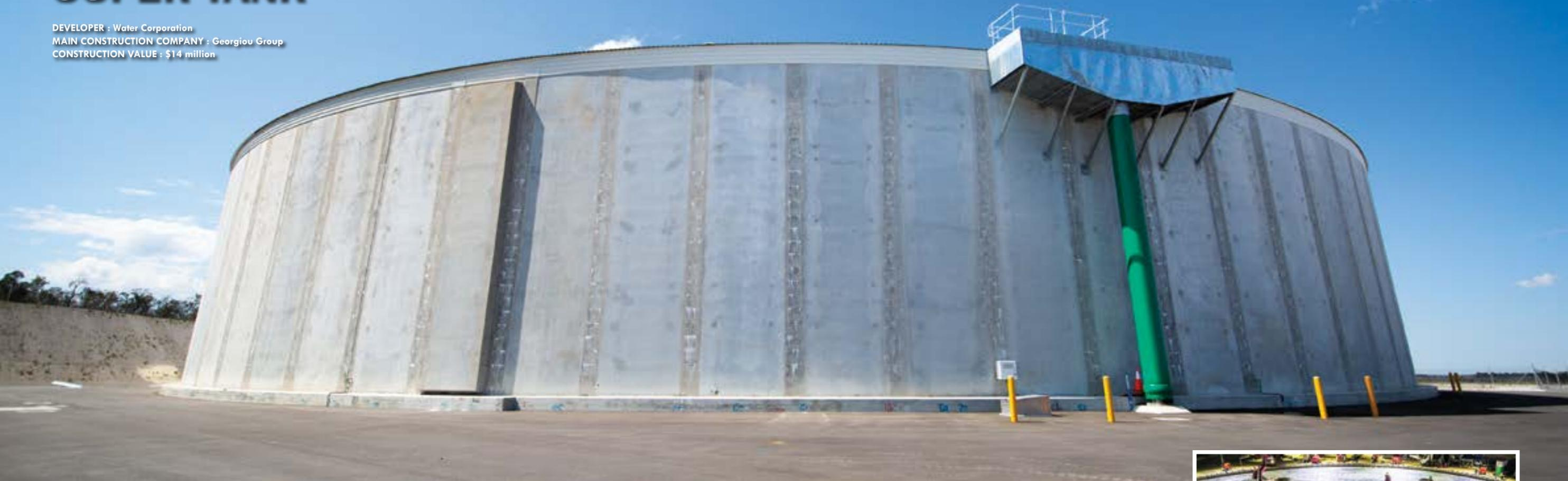
The 80 million litre Ellenbrook Tank, contains enough water to support the growth of Ellenbrook and the north eastern metropolitan corridor. Measuring approximately 90m in diameter and 14m in height it is the largest concrete tank Georgiou Group and the Water Corporation have ever constructed.
