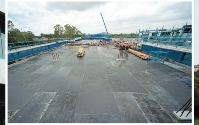
When it came to completing the formwork for the suspended slabs for BTP Northshore Hamilton, Trimform Pty Ltd used a combination of conventional formwork and Ischebeck formwork.
