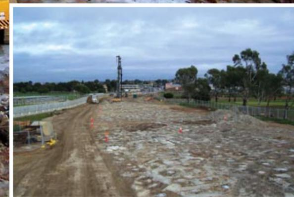
As part of the Breakwater Road upgrade, a new 800m long multi-span bridge has been built over the Barwon River and surrounding low lying area, which was prone to flooding. Geotechnical specialists Menard Bachy were brought in to address the low ground strength of the flood plain, where the new road was to be built and design and implement ground improvement, where necessary, to accommodate safely the bridge structure and daily traffic flow of around 20,000 vehicles.
