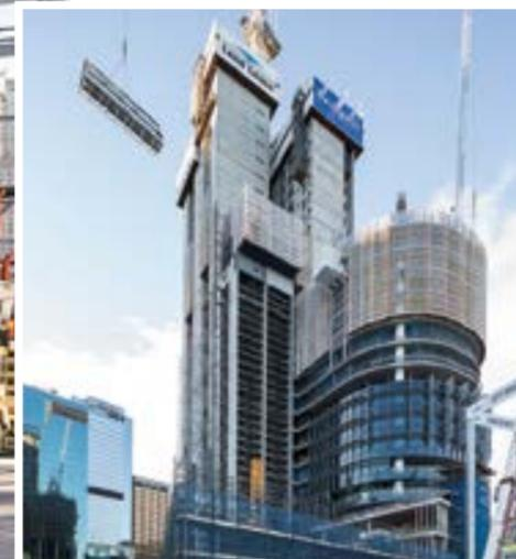
A.G. Coombs and Lendlease introduced a new way to install services risers – one that has not been applied before to very tall buildings in Australia. Ductwork, pipework, fire rated walls and platforms and other building services features have been pre-installed into engineered 3-storey frames in an off-site dedicated prefabrication factory.
