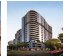
North Apartments North Melbourne
