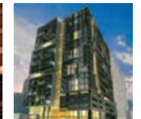
Guilfoyle Apartments South Melbourne
