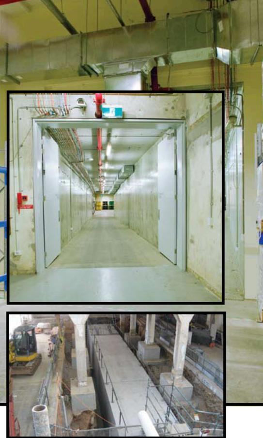
to get the shutters for the formwork in place, due to the limited height, which was only 4 metres of height inside the building, but there was a 7-metre trench to dig. Access was the biggest problem, as all the work had to take place inside the building, while the plant was still operational.
