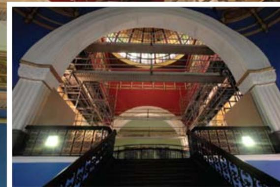
Instant Access was commissioned by head contractor, Built, to provide a specialist access solution to the internal atrium of the heritage listed Queen Victoria Building. Our scope of works was to provide access to the centre dome area as part of the refurbishment project to return the QVB to its former glory, with a new Victorian inspired color scheme more reflective of the original scheme when the QVB was first completed in 1898.
