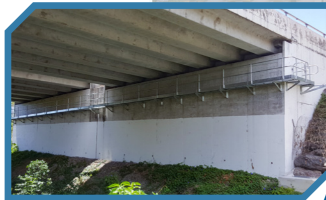
Transport for NSW, Yelgun Creek, twin bridge inspection platform.
