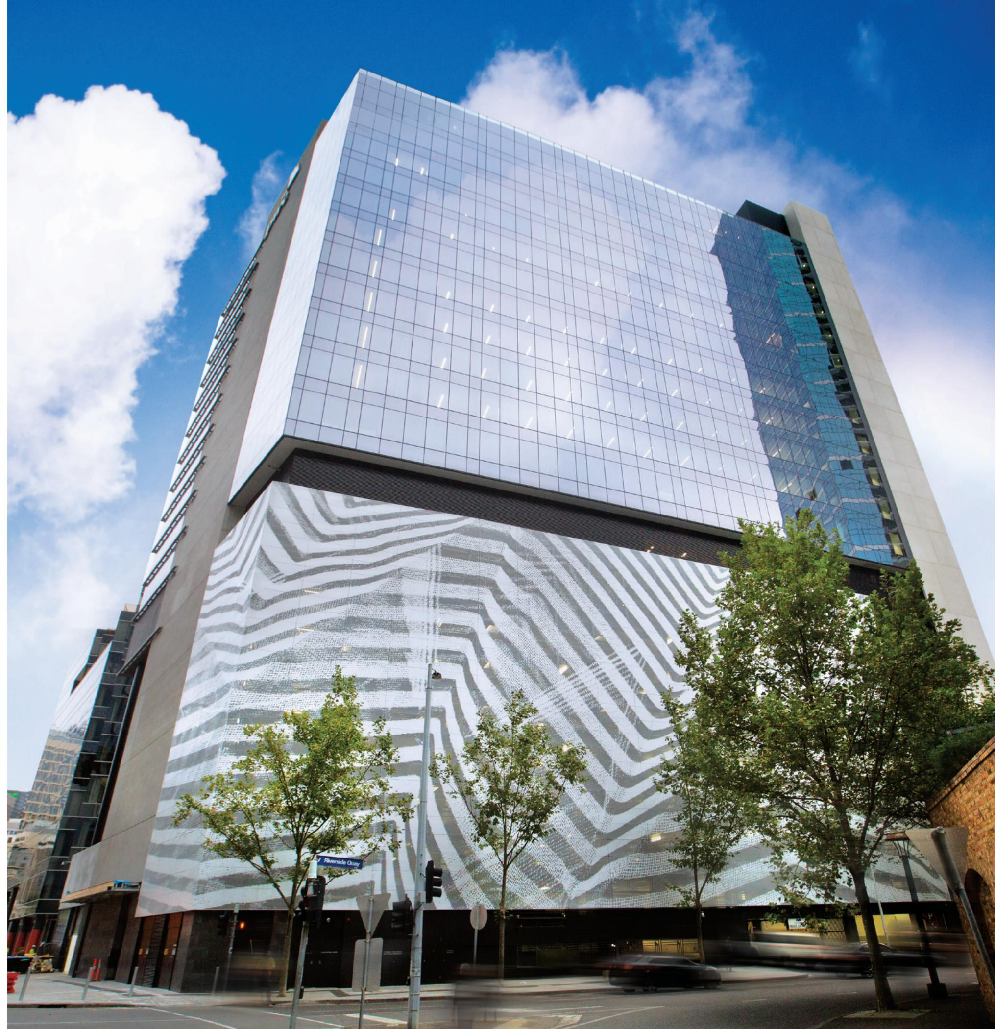
**Below** Custom Clad fabricated and installed 4,000m<sup>2</sup> façade panels for the 2 Riverside Quay project.
