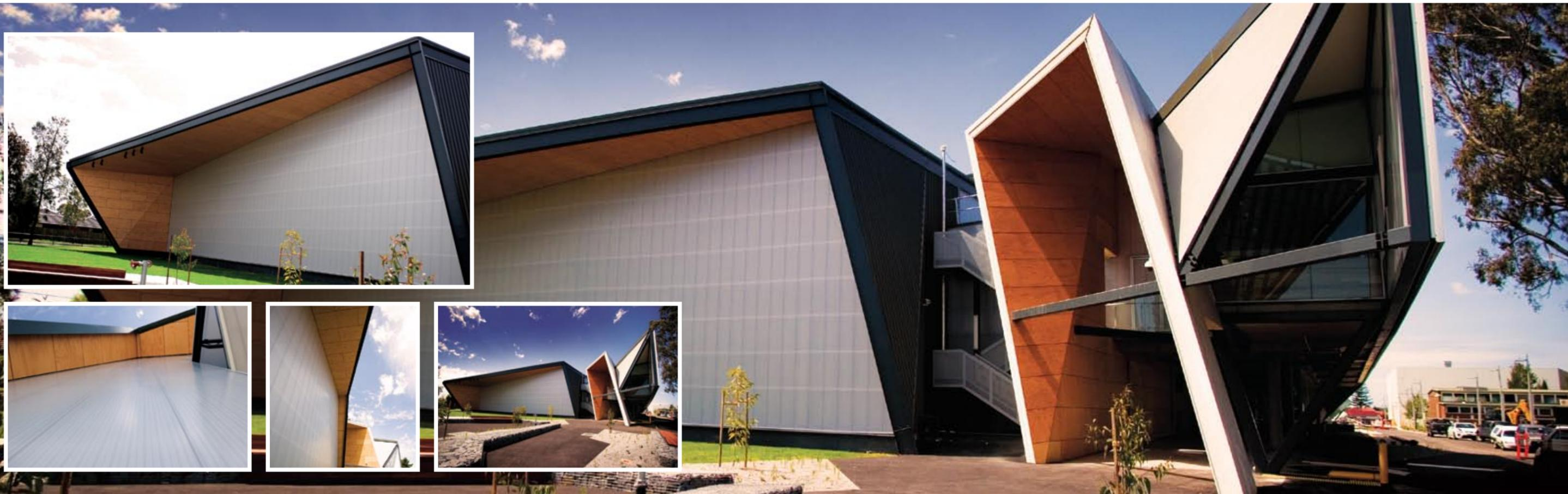
Nanokote was engaged to apply its EcoBarrier™ anti-graffiti coating to the Danpalon polycarbonate walls for the Victoria University Sunshine Construction Futures project. The Danpalon substrate was particularly susceptible to permanent damage from both graffiti markers and removal agents that would result in permanent damage to the surface.
