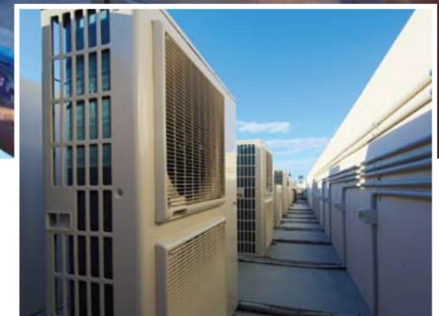
Acoustic considerations were paramount when locating plant. The location and treatment of noise-generating compressors, heat-rejection plant and fans were engineered to satisfy the strict requirements of the local council and Australian Standards.
