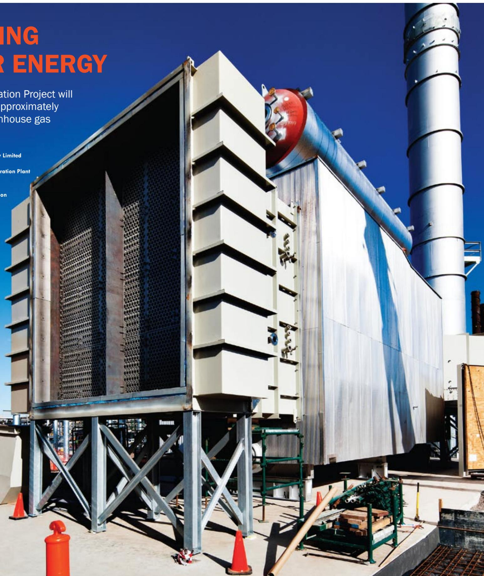
Left The cogeneration unit will be capable of producing over a third of its steam requirements and will meet all of Qenos's electricity demands.
