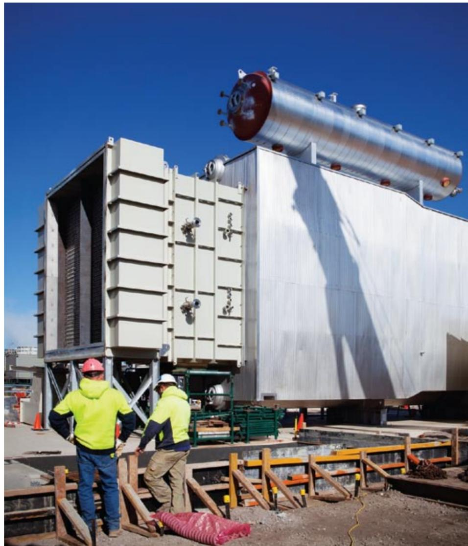
Below Accord Logistics (Aust.) were contracted by UGL to transport the Heat Steam Recovery Generator onto the foundation at the Qenos Cogeneration Plant.
