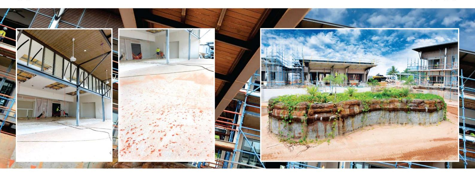
Darwin-based company JGA Concreting was responsible for the preparation of concrete works on the SKYCITY Beach Resort. This involved minor formwork, sand filling, placement of mesh,
