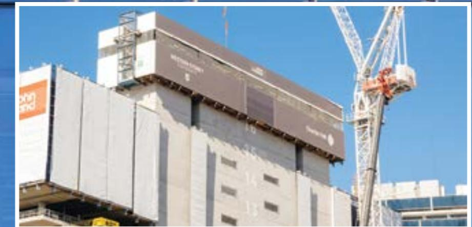
**Strategic Formwork entered the Australian market in 2002, with its inhouse designed and developed self-climbing 'CoreMaker' jumpform system for the construction of core vertical elements.**
