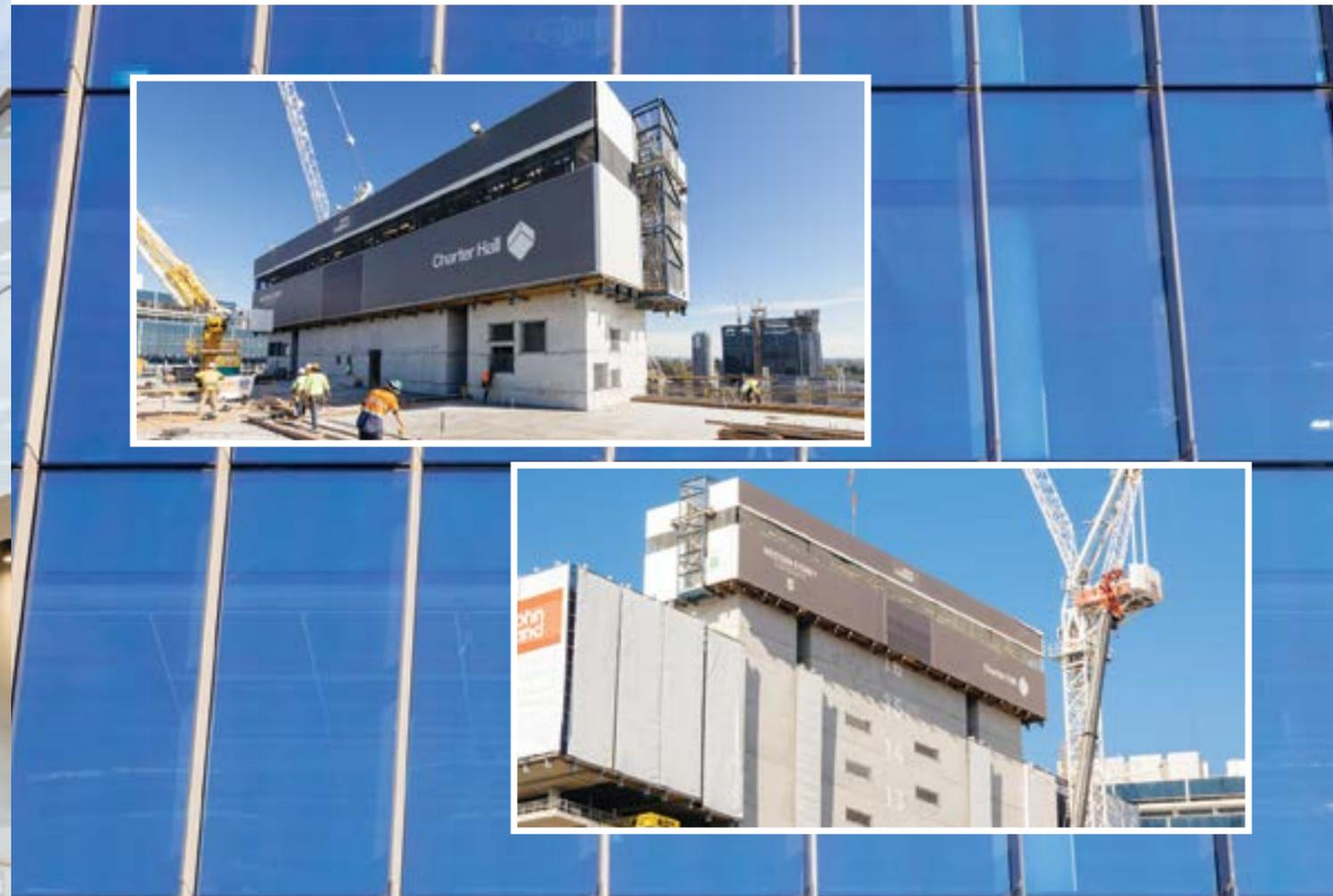
**Strategic Formwork entered the Australian market in 2002, with its inhouse designed and developed self-climbing 'CoreMaker' jumpform system for the construction of core vertical elements.**
