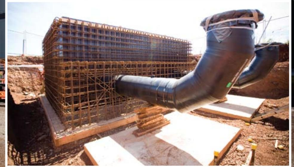
Over a period of 18 months, Pipecon installed 30km of 800mm diameter GRP for the Melbourne to Geelong Pipeline, stretching from Tarneit to Little River. It was not an easy task, with the challenges including two open cut river crossings, demanding timeframes and high quality expectations.
