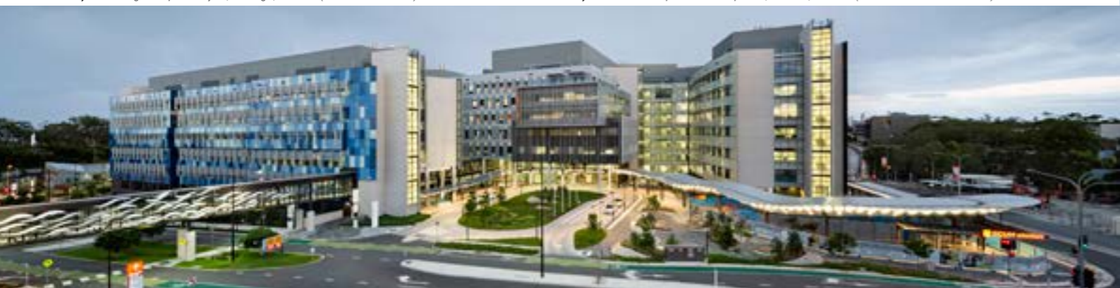
Project: Gold Coast University Hospital, Southport, Queensland (STH+PDT+HASSELL)
