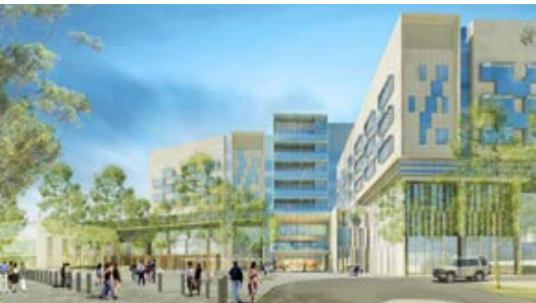
Project: Bendigo Hospital Project, Bendigo, Victoria (STH+Bates Smart)
