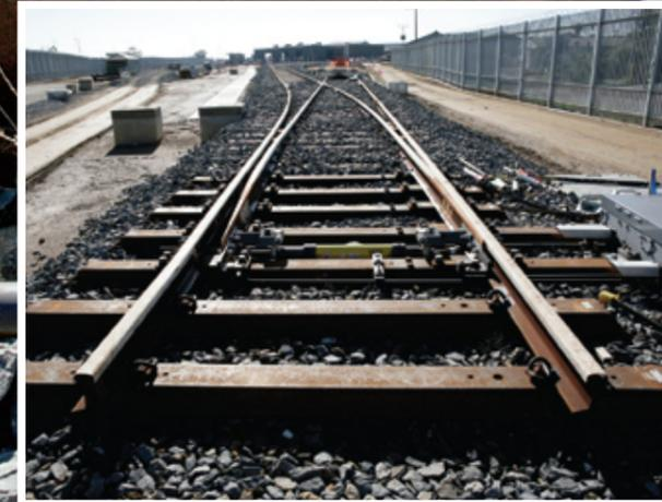
**V**AE Railway Systems Pty Ltd (Australia) were commissioned to provide turnouts and associated high technology rail-line devices for the 11 kms of trackwork specified for Adelaide's new Dry Creek Railcar Depot.
