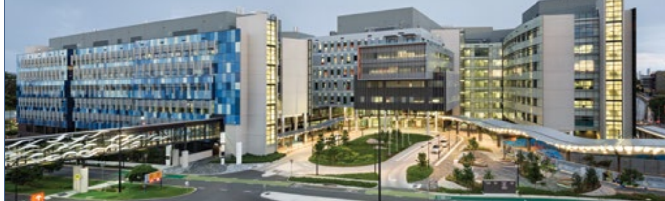
Gold Coast University Hospital Joint venture with PDT and Hassell Architects
