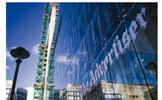
two layers of glass in the façade is a 1-metre wide walkway to enable cleaning.
