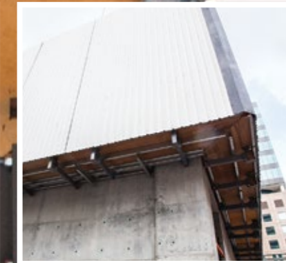
ABOVE: Sureform's Self-climbing formwork system at 35 Albert Road for E-Form P/L
