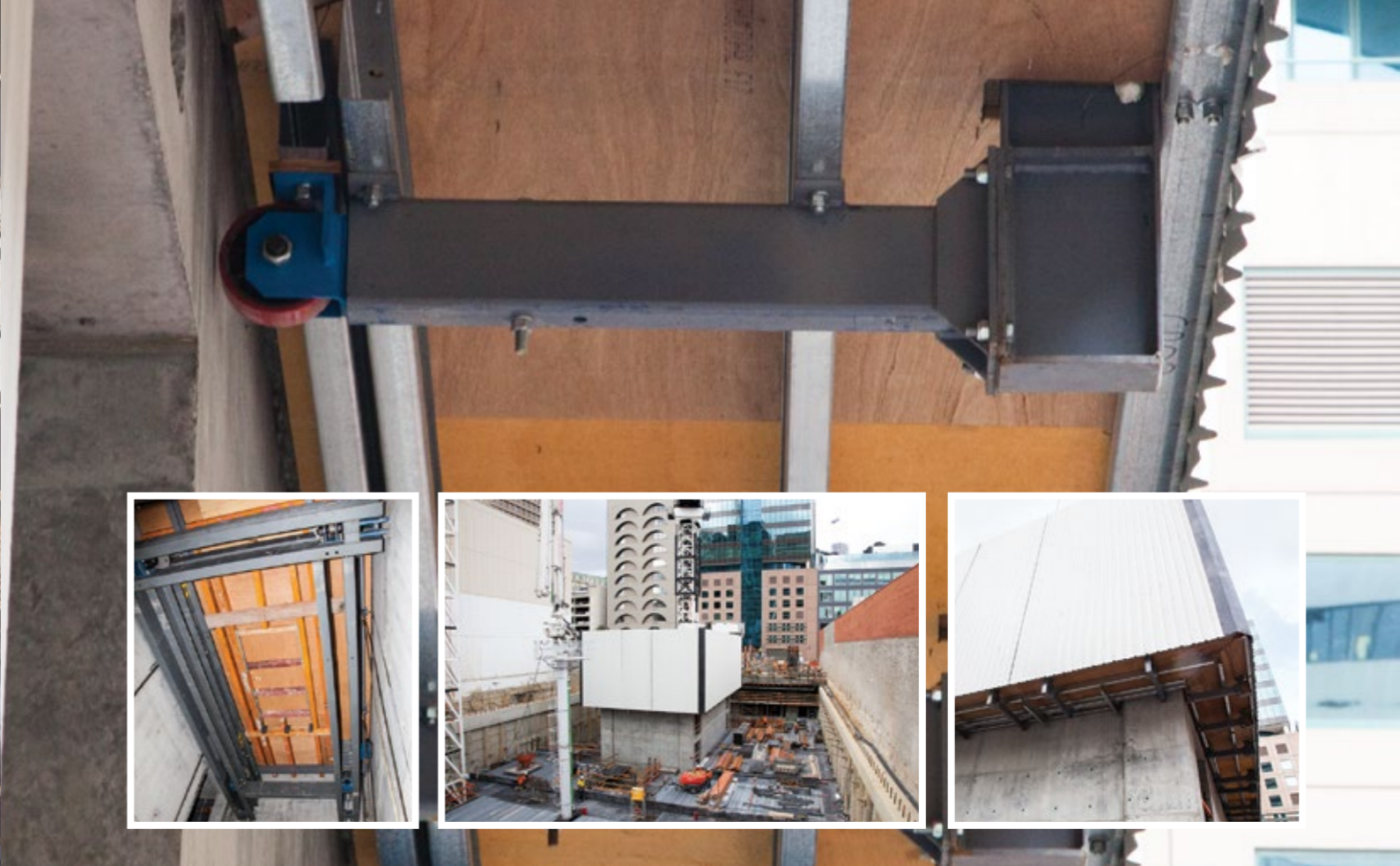
ABOVE: Sureform's Self-climbing formwork system at 35 Albert Road for E-Form P/L
