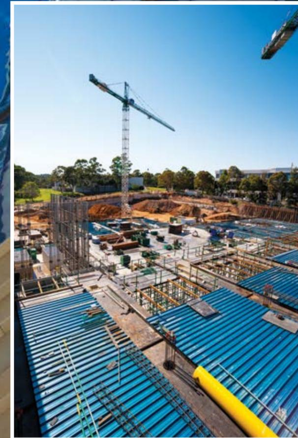
**De Martin and Gasparini (DMG) were awarded the contract for all in-situ concrete works required for the 161 Castlereagh Street, Sydney project.** The scope included the supply, pump, place and finish of approximately 36,000m<sup>3</sup> of concrete. The project brief required the supply and delivery of high strength, high performance 'green' concrete, having no less than 20% cement and 20% aggregate replacement, without compromising structural integrity.
